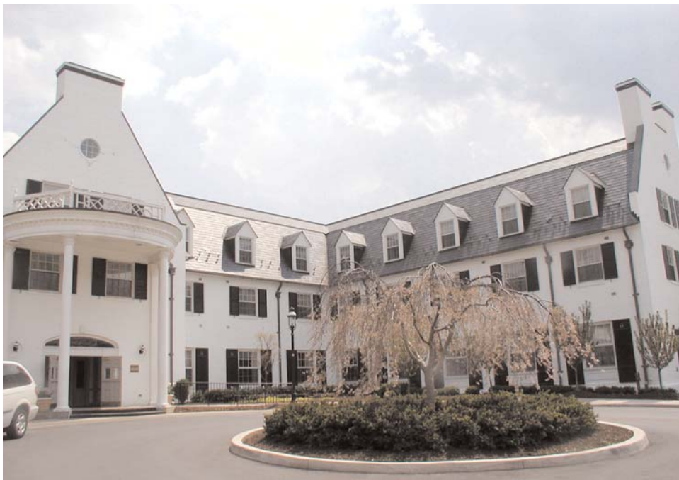
Nittany Lion Inn. Photo by Chris Koleno, Penn State Department of Public Information.
